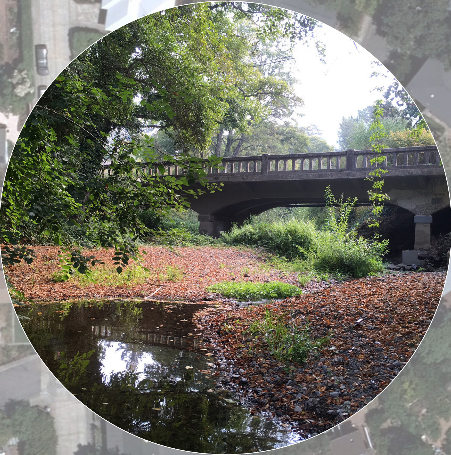
View of Bridge from West
